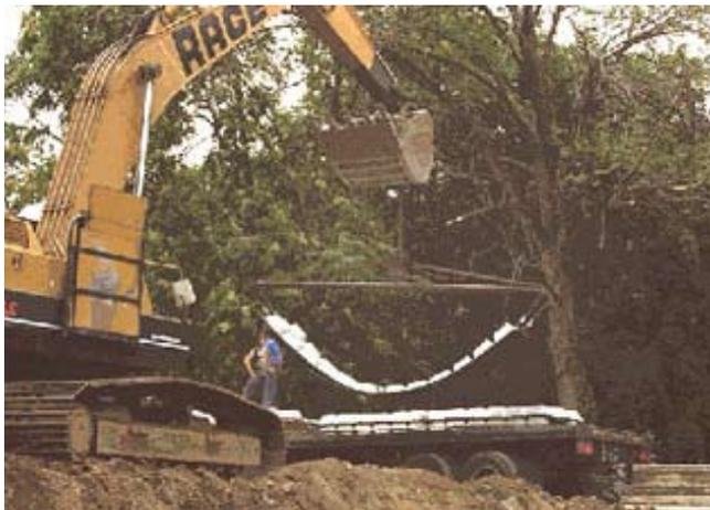
**Figure TS14L-19** Hand placement of ACB blocks
